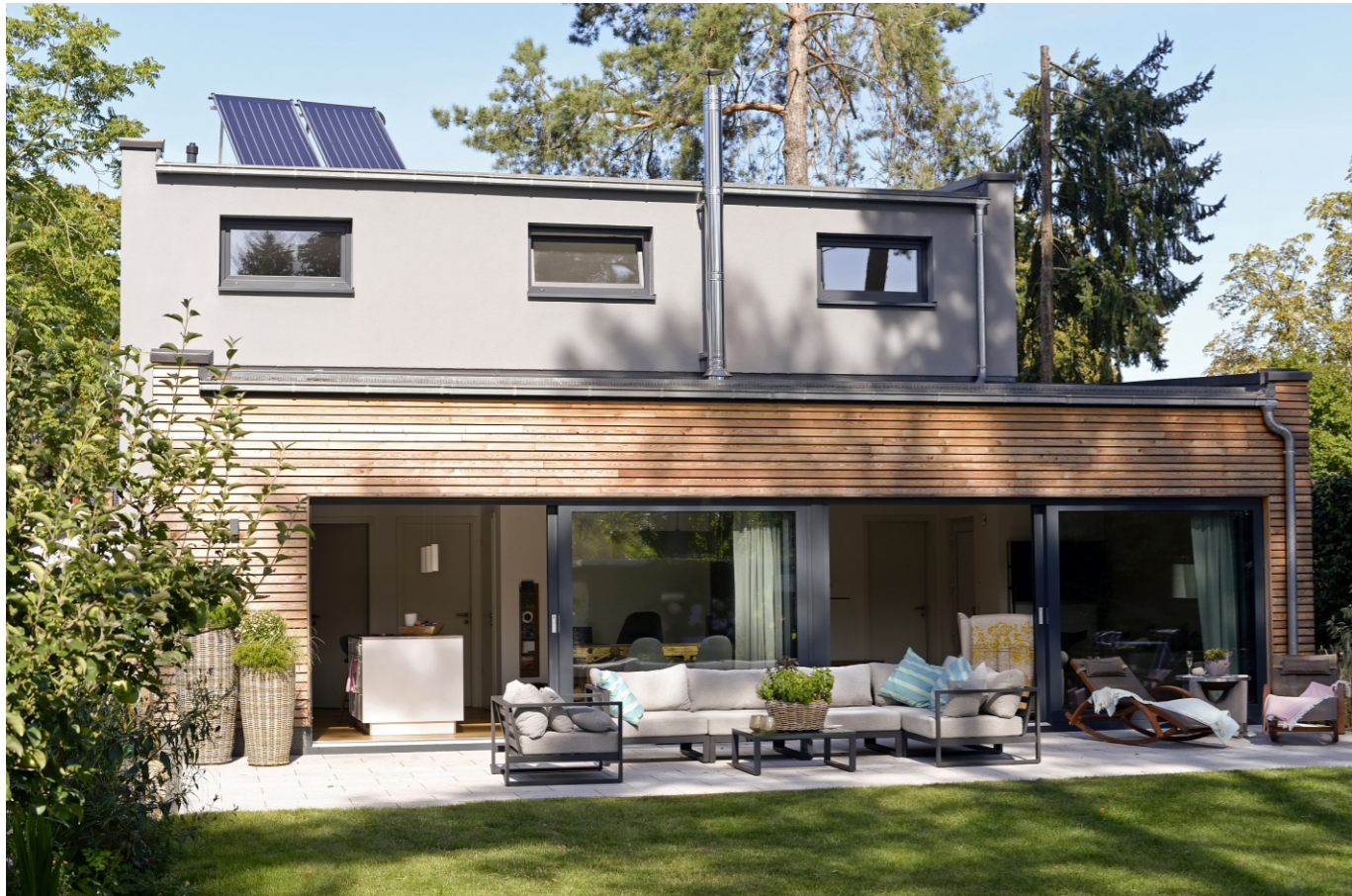
Solar Home System
