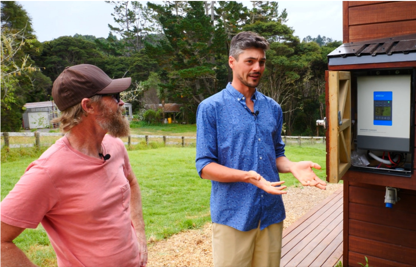
Solar Home System
